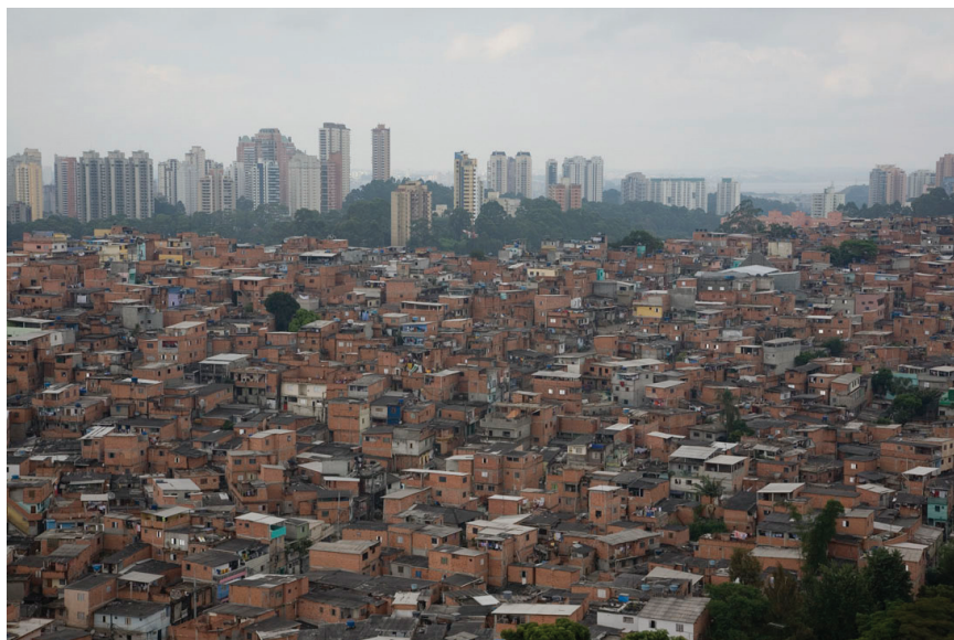
FIGURE 2-4 Juxtaposition of urban slums and modern buildings in São Paulo, Brazil. SOURCE: Image courtesy of Zema Fontoura.
